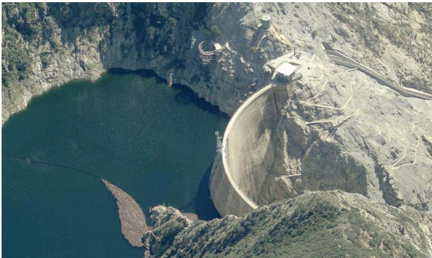
Figure 8-29 Photo of Pacoima Dam
