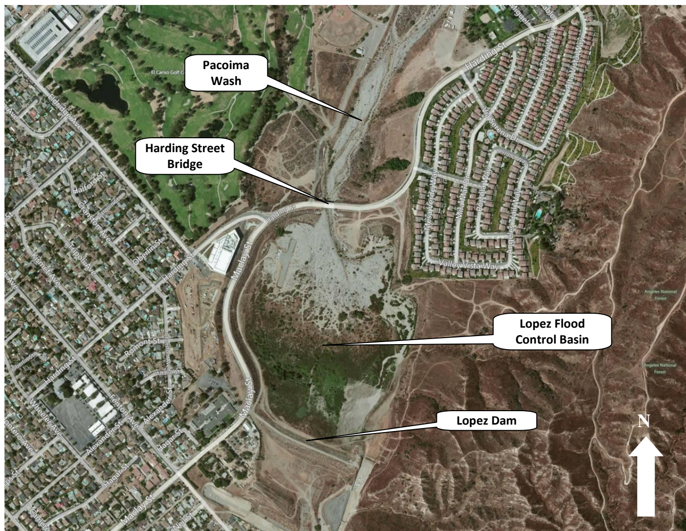
Figure 8-34 Lopez Flood Control Basin
