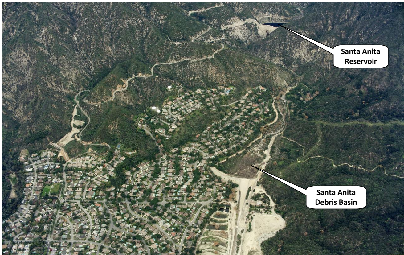
Figure 8-79 Santa Anita Debris Basin
