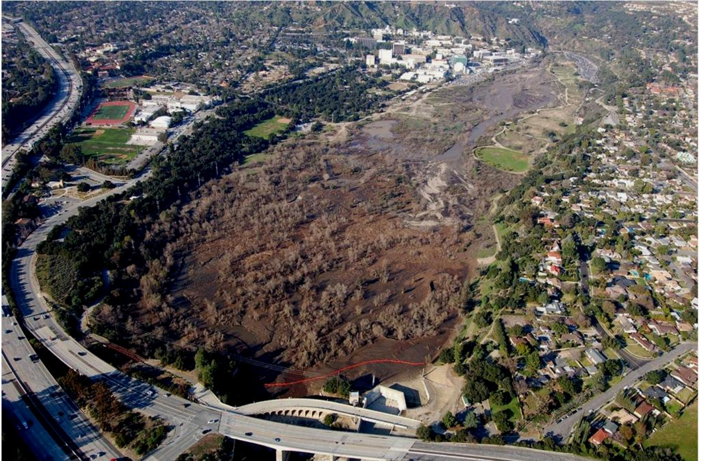
Figure 8-24 Aerial of Devil’s Gate Reservoir
